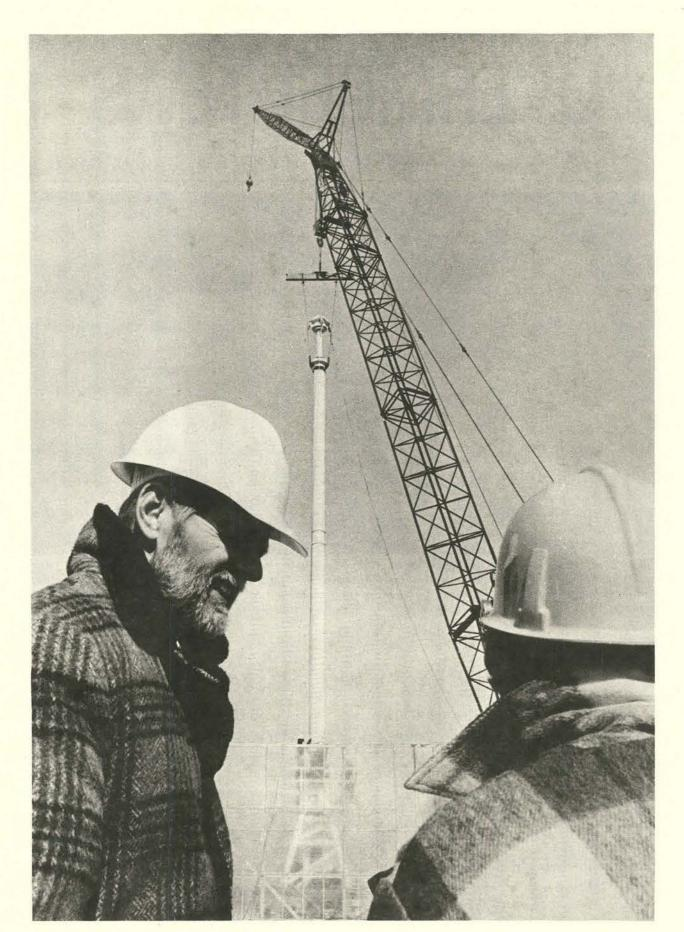
NEW WIND TURBINE SHAFT, is emplaced on a 5.5 m base east of Area I. With the anemometer tower added later, total height is 33.5 m. The revolving shaft will eventually support three experimental blades (arranged to form a 17 m diameter sphere) and drive a generator. Here Bob Grover and Carl Longfellow (both 5715) debate the delights of riding a crane-lifted cage to bolt on the anemometer tower. (Both lost out to Ralph Rusk, also 5715.)
